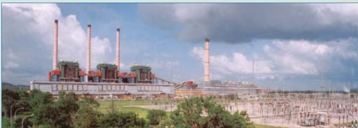
500 MW Unit-7 at Ramagundam STPS synchronised in a record time of 36 months & 10 days
