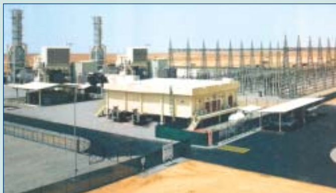
Qarn Alam Power Project of Petroleum Development Oman, equipped with first-ever Advanced-Class GTGs (2x70 MW ISO), exported from India
