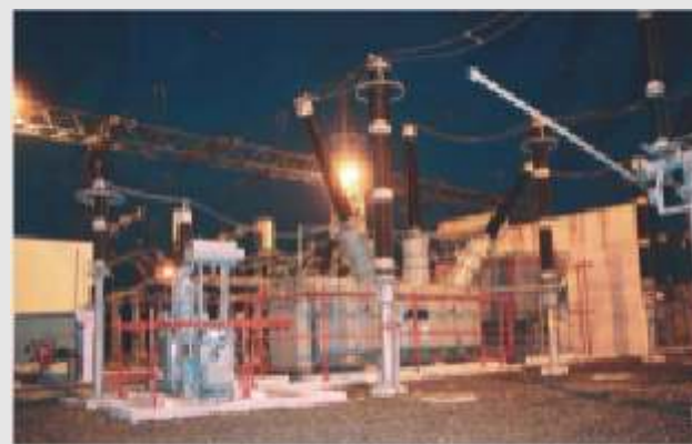
The first-of-its-kind in the world, Controlled Shunt Reactor (CSR) developed In-house by BHEL
