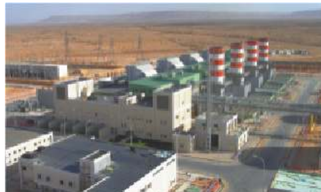
600 MW Western Mountain Power Project in Libya
