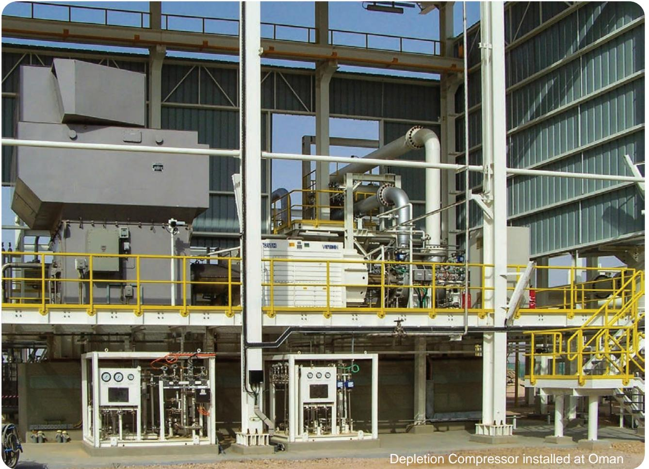
Depletion Compressor installed at Oman
