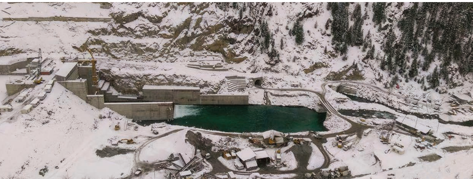
3x110 MW Kishanganga Power station in Jammu & Kashmir, India, commissioned by BHEL
