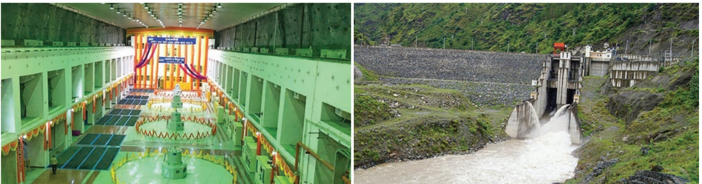
Exterior view of (Inset: Generator floor) 4 x 130 MW Parbati-III HEP, NHPC Ltd. In Himachal Pradesh, India
