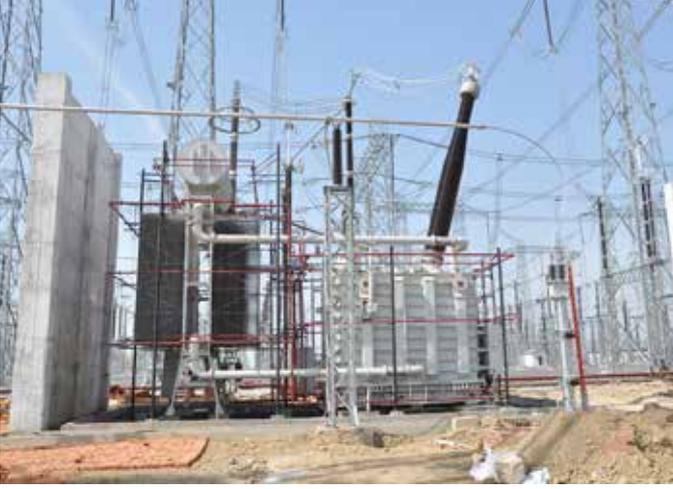
India's first 400 kV Controlled Shunt Reactor at Itarsi Substation
