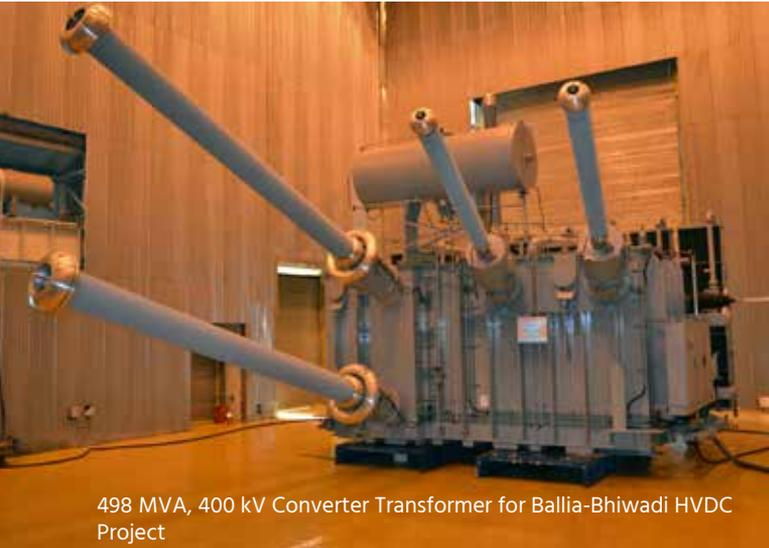
498 MVA, 400 kV Converter Transformer for Ballia-Bhiwadi HVDC Project
