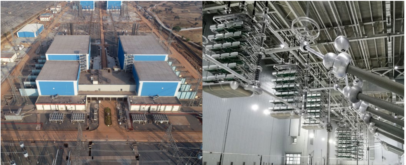
Aerial view and HVDC hall of Raigarh substation of the \pm 800 kV, 6000 MW Raigarh-Pugalur HVDC link commissioned by BHEL
