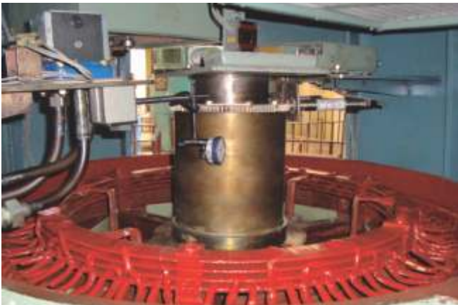
Brushless Exciter developed at BHEL's R&D Centre installed at Devighat HEP, Nepal
