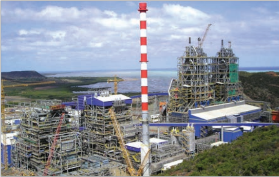
2x135 MW Circulating Fluidised Bed Combustion Boilers under commissioning at New Caledonia
