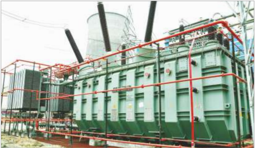
India's first Phase Shifting Transformer developed & manufactured by BHEL, installed at Kothagudem
