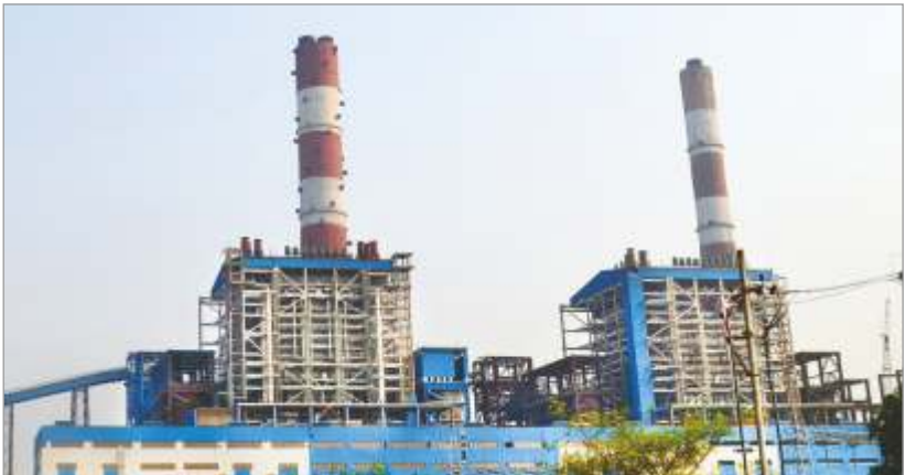
Indigenously manufactured supercritical set of 660 MW rating commissioned by BHEL at Barh 5
