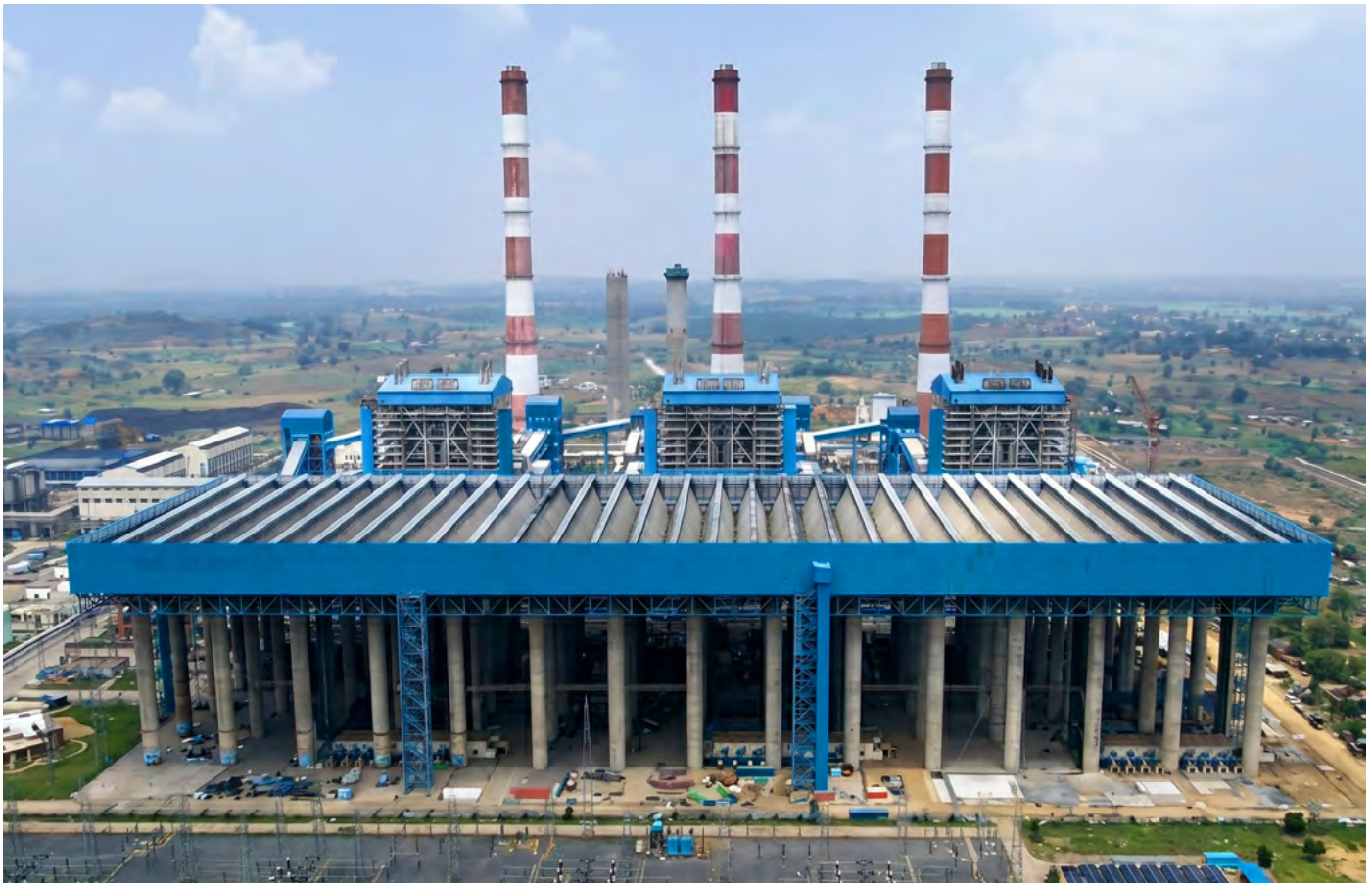
3x660 MW North Karanpura Super Thermal Power Project, located in Jharkhand, commissioned by BHEL. Notably, this is India's first large-scale supercritical thermal plant equipped with a direct Air Cooled Condenser (ACC)
