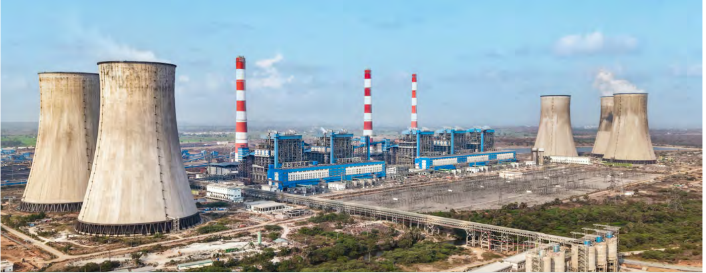
Full load achieved for Unit# 3 of 5x800 MW Yadadri Thermal Power Station in Telangana
