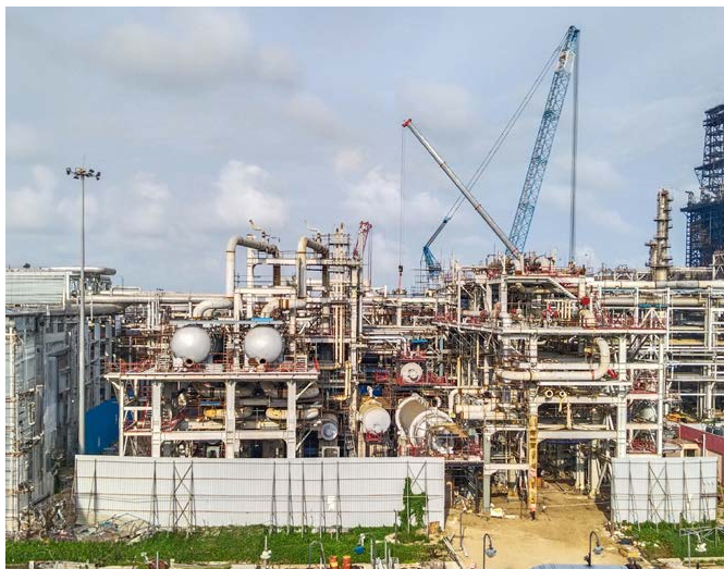
Sulphur Recovery Unit (SRU) project under execution at IOCL Paradip, Odisha
