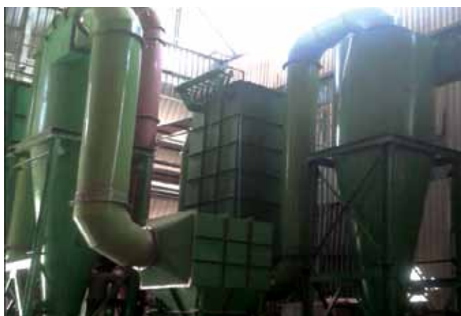
New dust extractor system equipped with spark arrestor at HEP Bhopal
