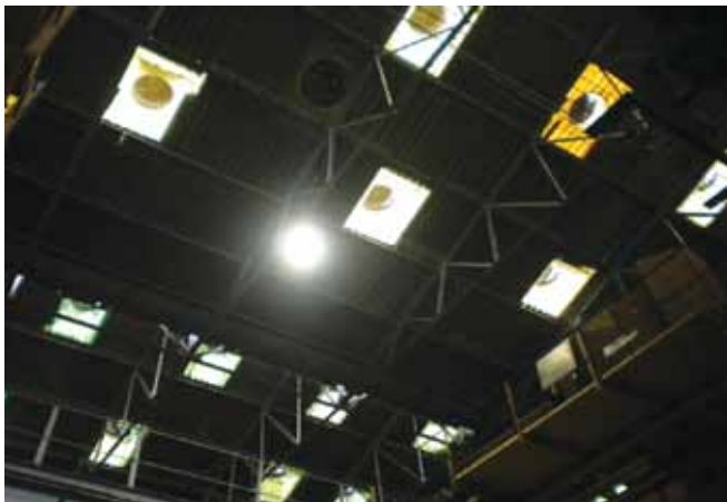
Introduction of fume extractors in the heat treatment and surface treatment areas for sending out the toxic fumes at HPEP Hyderabad Unit
