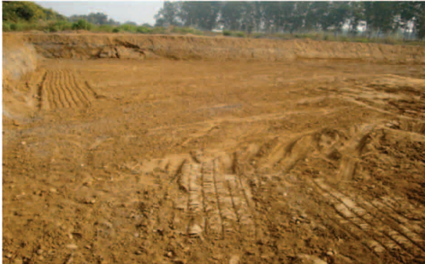
Earthen pond for storm water retention under construction, Haridwar
