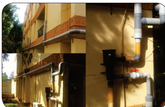
Rooftop Rainwater Harvesting at EPD Bangalore
