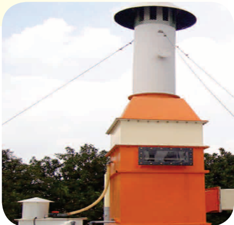
New Scrubber erected at ACID Texturisation System for washing the exhaust mist at EDN Bangalore
