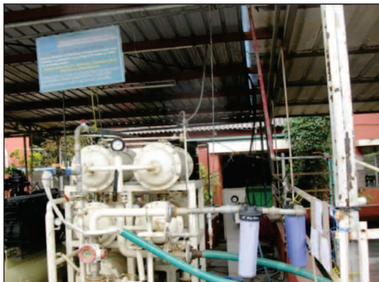
Ceramic membrane based micro filtration ~ 200 nm – Reuse of Waste Water at EPD – Bangalore
