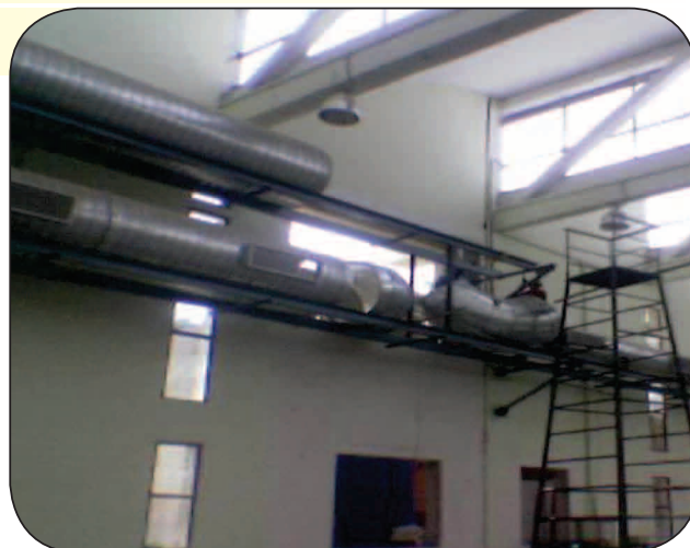
Effective utilization of day light by using light efficient (Ultra-violet stabilized )poly carbonate sheets in north lighting at EDN Bangalore
