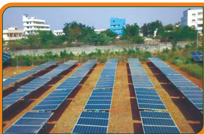
BHEL has successfully developed and demonstrated 50kWp SPV systems using sun trackers based on liquid balancing system
