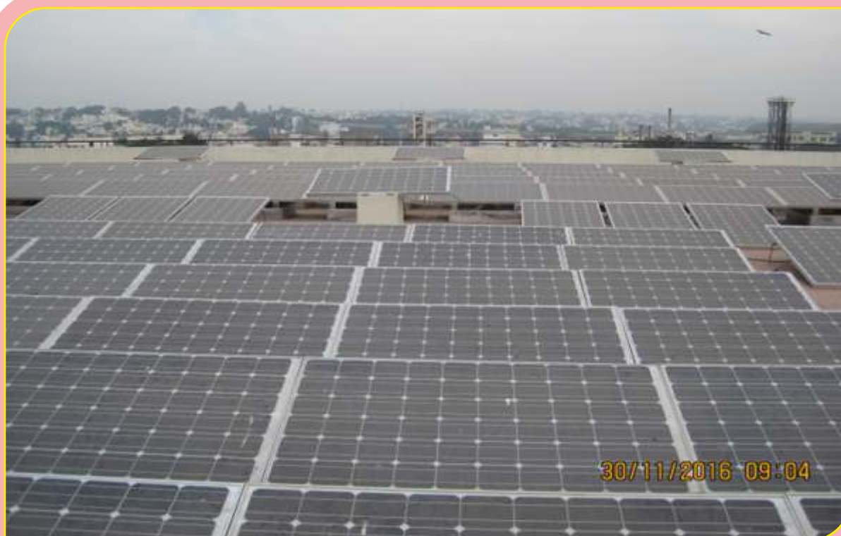
60 KWp Photo- voltaic panels mounted on New Engineering Building at EDN Bengaluru
