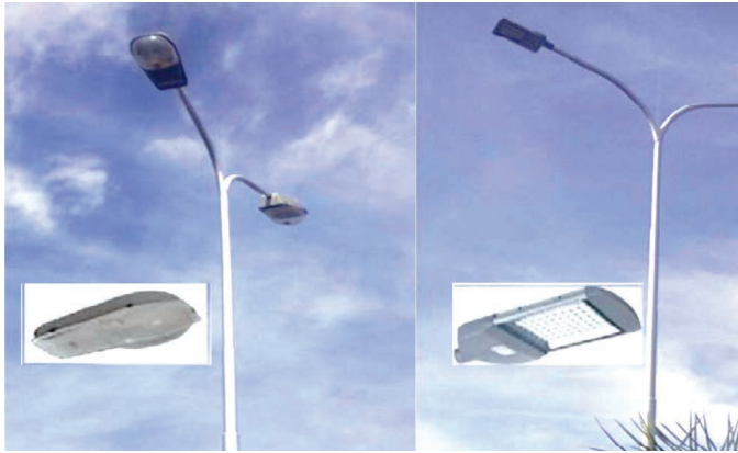
Figure 38: Replacement of 150 W Sodium Vapour light with 60 W LED Fittings on trial basis at Trichy unit
