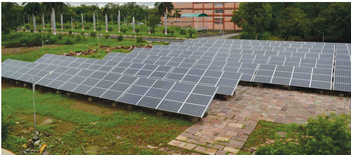
Figure 37: 250 kW p Grid interactive Solar Power Plant installed at HEP Bhopal unit
