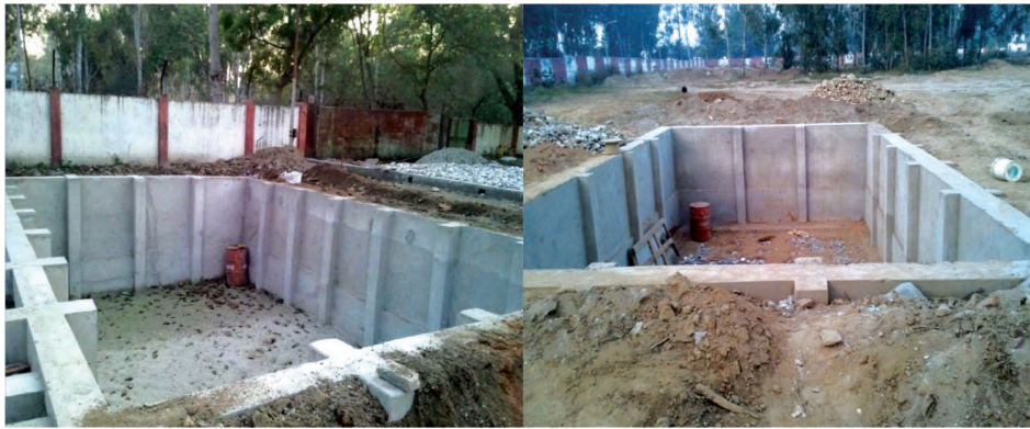
Figure 45: 6mX10m and 5mX10m Rain Water Recharging pits inside factory premise at HEEP Haridwar
