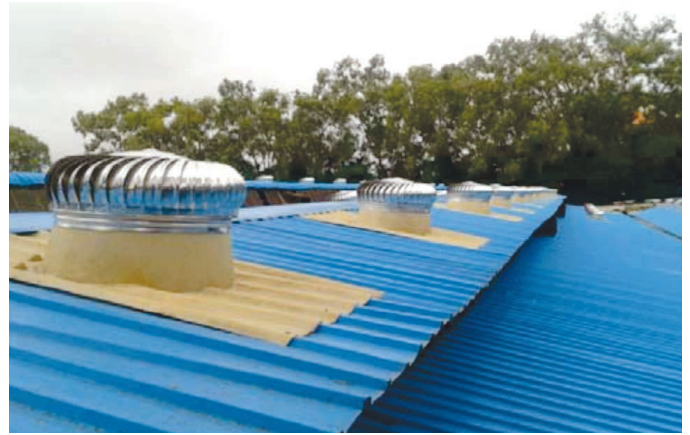
Figure 39: Turbo ventilators installed at EPD Bangalore
