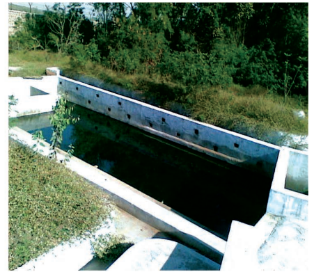
Figure 46: Rain water harvesting pit inside factory premise at Jhansi
