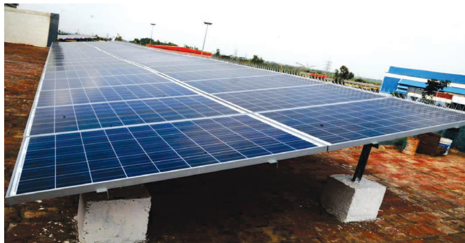
Figure 37: 250 kW p Grid interactive Solar Power Plant installed at HEP Bhopal unit
