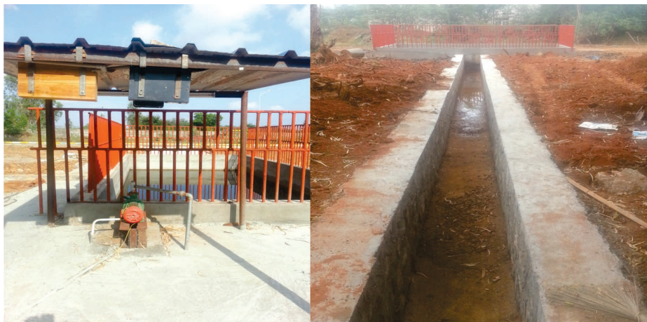
Figure 48: Rain water harvesting sump connected through channel with pumping arrangement for using the rainwater collected for gardening purpose inside factory premise
