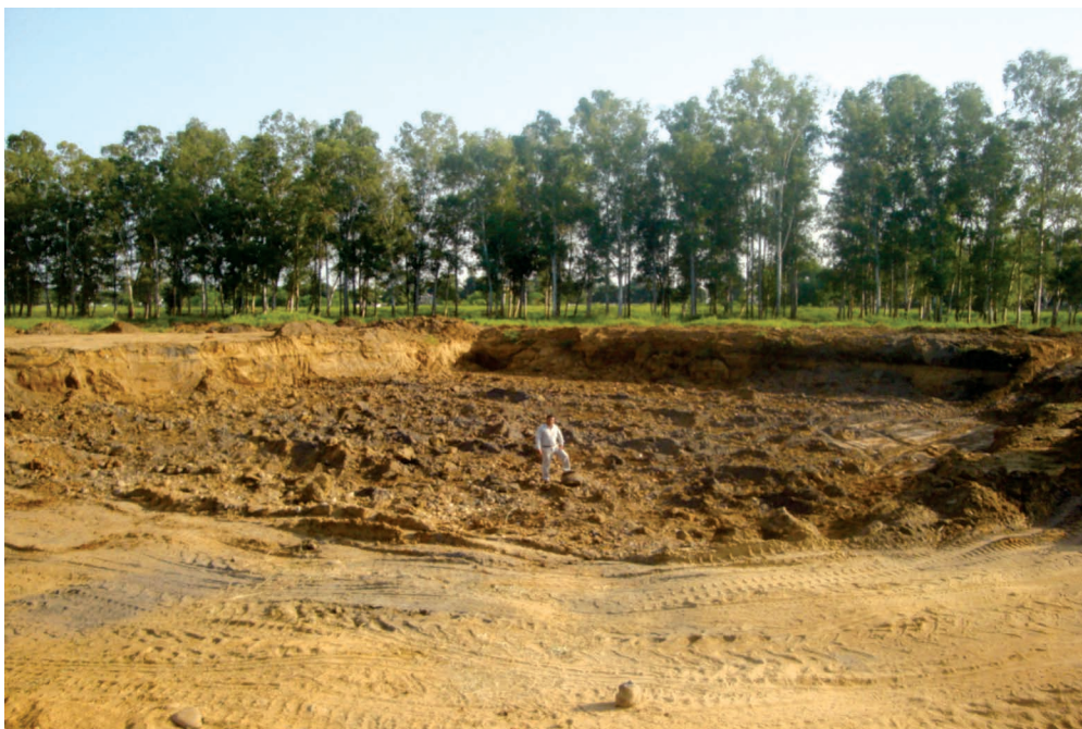
Figure 45: 6mX10m and 5mX10m Rain Water Recharging pits inside factory premise at HEEP Haridwar
