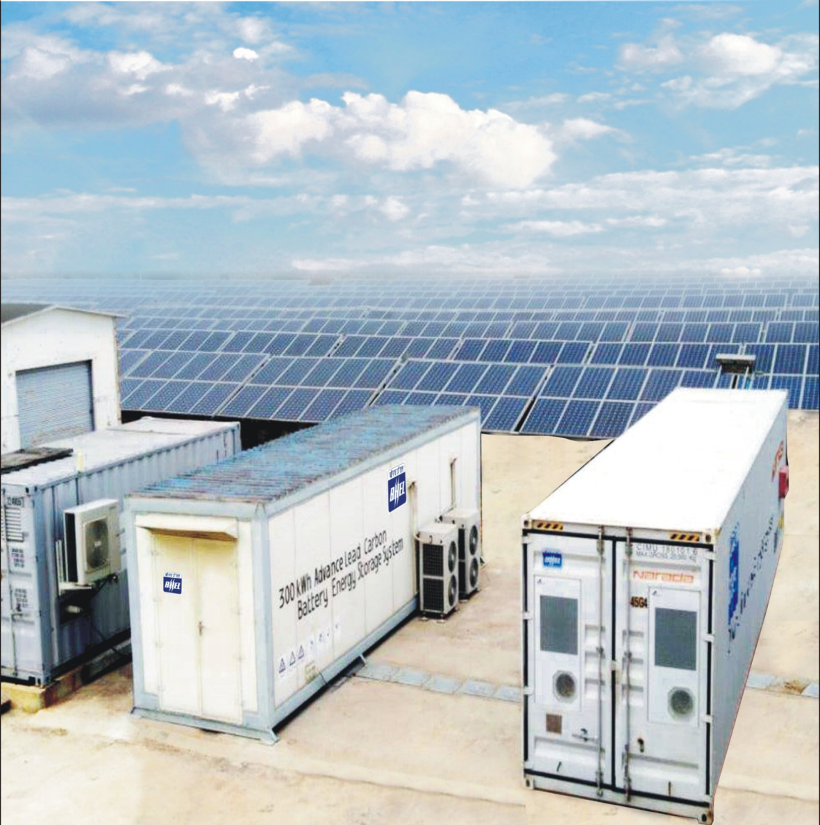
1 MWh Grid Connected Battery Energy Storage System (BESS) installed at BHEL Corp R&D
