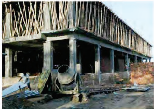
Construction of Tribal Welfare School in Bhubaneswar Nagar, Assam
