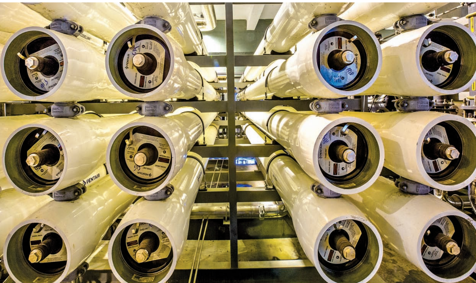
RO membranes of RODM Plant at RPCL Yerammaru, commissioned by BHEL
