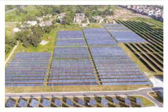
5 MW solar power plant including ground mounted, fixed, motor tracking & passive tracking enabled modules of BHEL make at Haridwar plant premises
