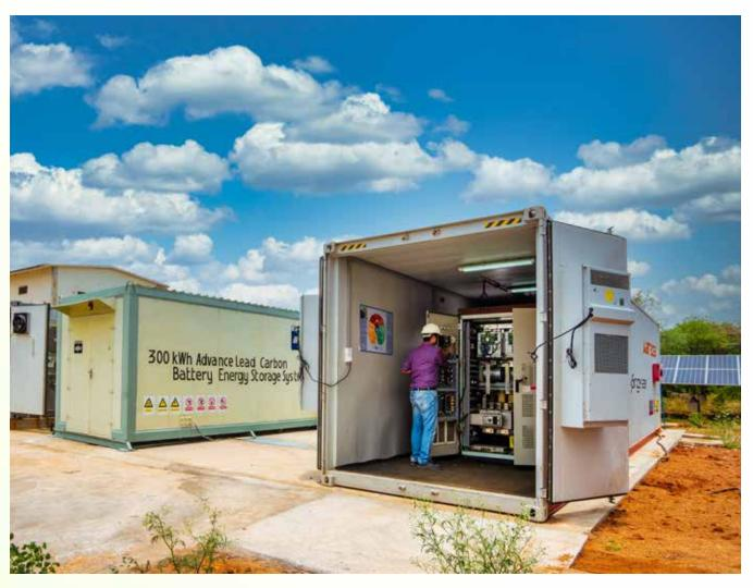
1MW Battery Energy Storage System (BESS) for in-house usage, developed & commissioned at Corporate R&D, Hyderabad
