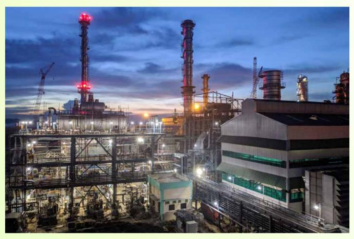
RFCL Ramagundam CPP with 32.5 MW rating Gas Turbine along with Utility Boiler and Heat Recovery Steam Generator under commissioning by BHEL in Telangana
