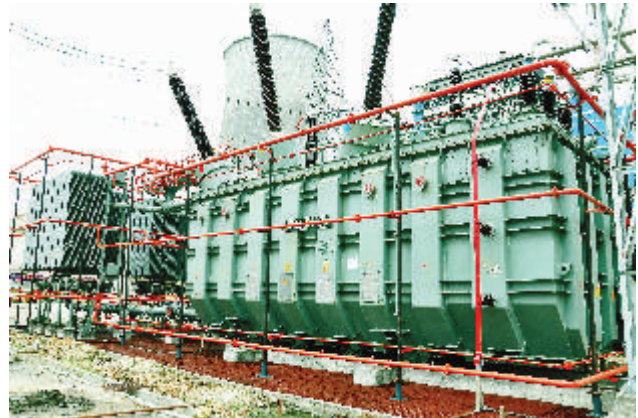
India's first 400 kV Phase Shifting Transformer
