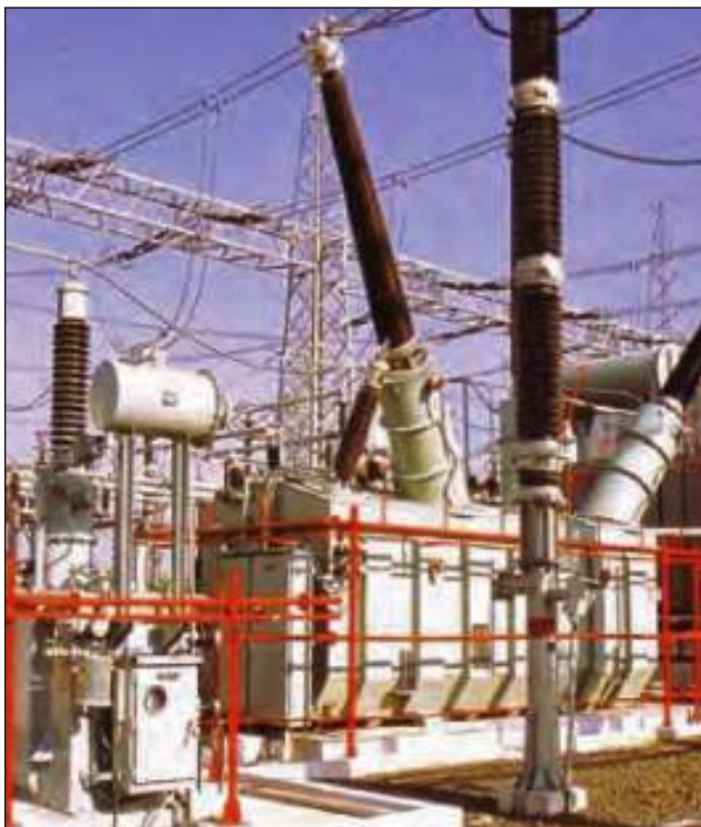
India's first 400 kV Controlled Shunt Reactor at Itarsi Substation
