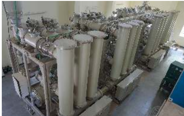
BHEL make 145kV GIS at Vittalwadi Substation
