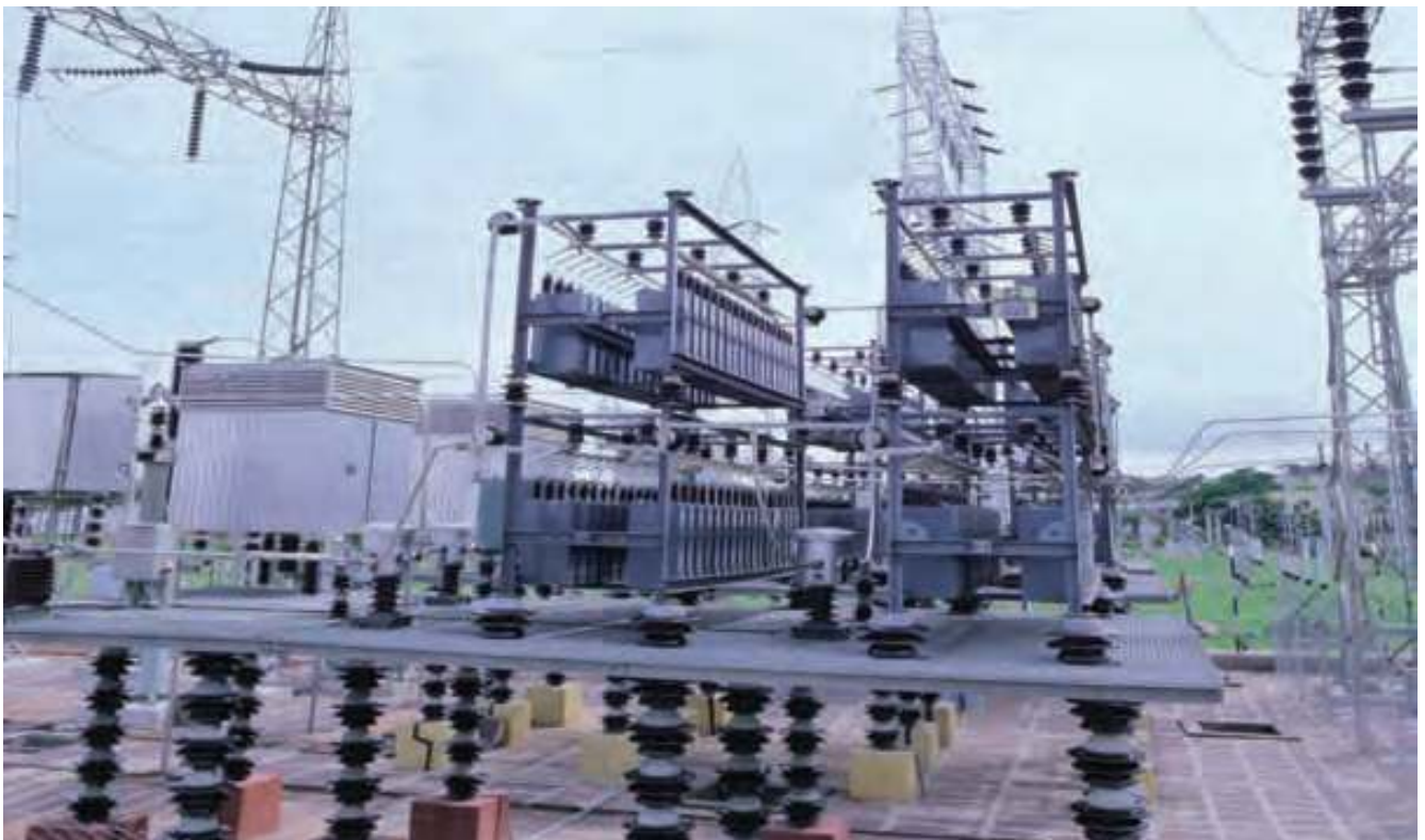
Fixed Series Compensation Scheme at Ballabhgarh
