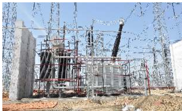
80 MVAR, 765 kV shunt reactor at Greater Noida Substation
