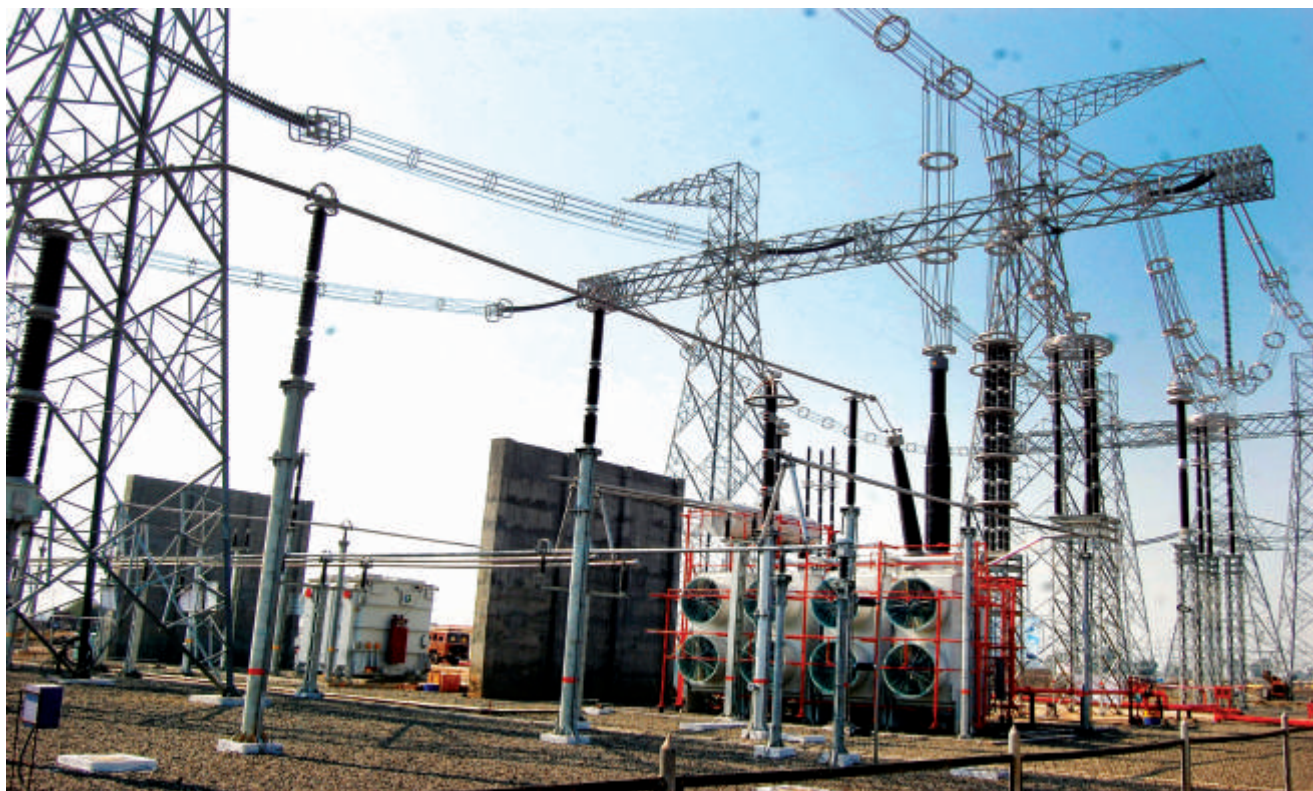
Country's first 1200kV power transformer at PGCIL's Bina test station
