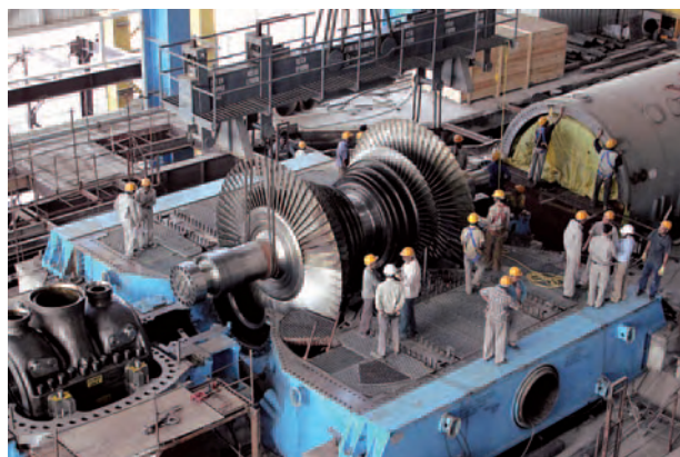
500 MW TG set under erection at 3x500 MW Indira Gandhi STPP at Jhajar
