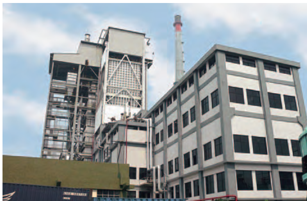
Captive power plant of PT- Indo Bharat Rayon, Indonesia - comprising 1X15 MW STG & 120 TPH CFBC boiler
