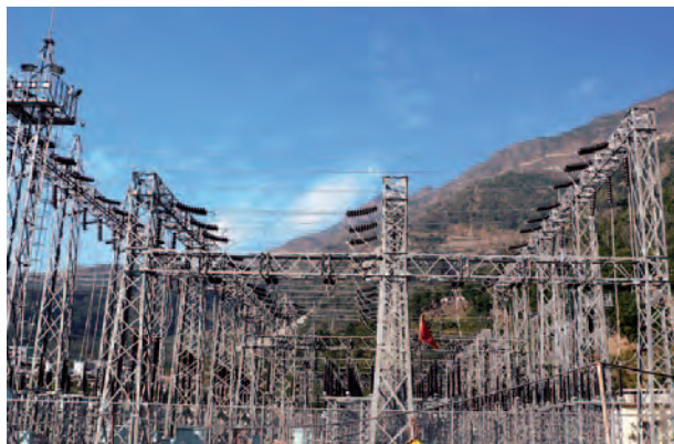
132 kV Switchyard of Sewa HEP
