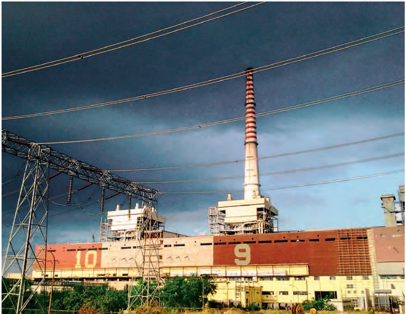
2X120 MW (Unit 9 & 10) of NALCO Captive Power Plant. With this BHEL has executed 10 units of 120 MW each in a single location
