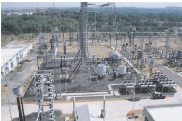
DC switchyard of 200 MW, \pm 500KV HVDC Project
