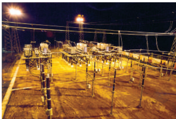
Series Compensation Scheme installed in 400 KV Kanpur-Ballabgarh transmission line of PGCIL
