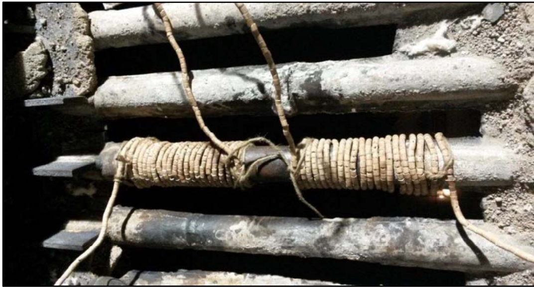
Figure B3.1: Preheating by Resistance coil winding
