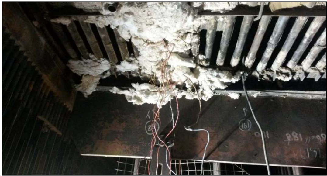
Figure B3.6: PWHT in progress
